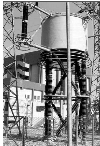
FIGURE 24.8 Installation of an air-cooled smoothing reactor.
